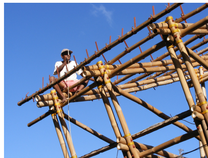
Fig. 17 -Constructing the Millennium school.
